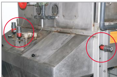
Sludge thickening process: Bearing lubrication at excess sludge densifier
