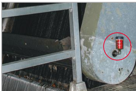
Screening: Lubrication of chain guide rollers
