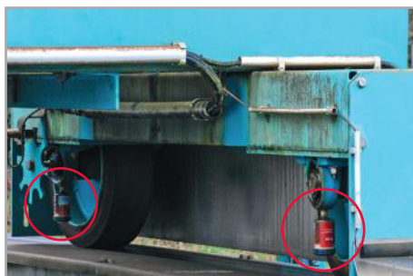
Clarifier tank: Bearing lubrication at the wheel of the circular scraper
