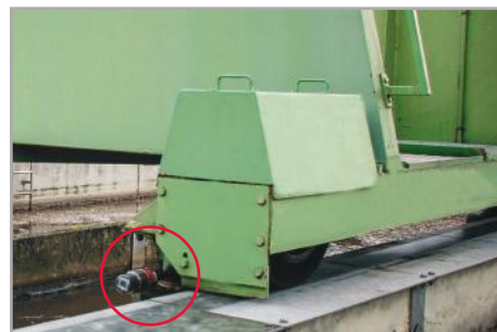
Primary sedimentation tank: Lubrication of impeller wheel bearing
