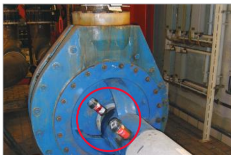
Lubrication of drive shaft on a pump
