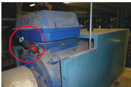
Lubrication of pump motor
