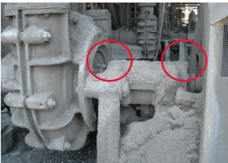
Pumps are normally operated under extreme conditions. These can include **heavy contamination** from slurry or dust and **hazardous materials** such as alkali solutions and weak acids.
