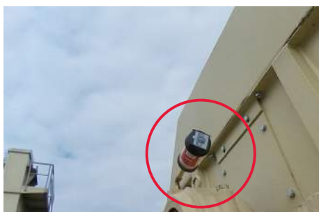
Pillow block lubrication on an RA-Elevator
