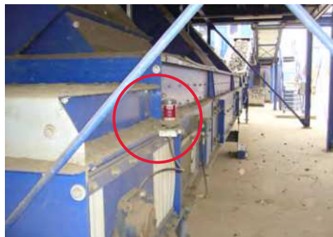
Flange bearing lubrication on a conveyor
