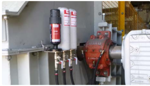
Conveyor pulley bearings and seals
